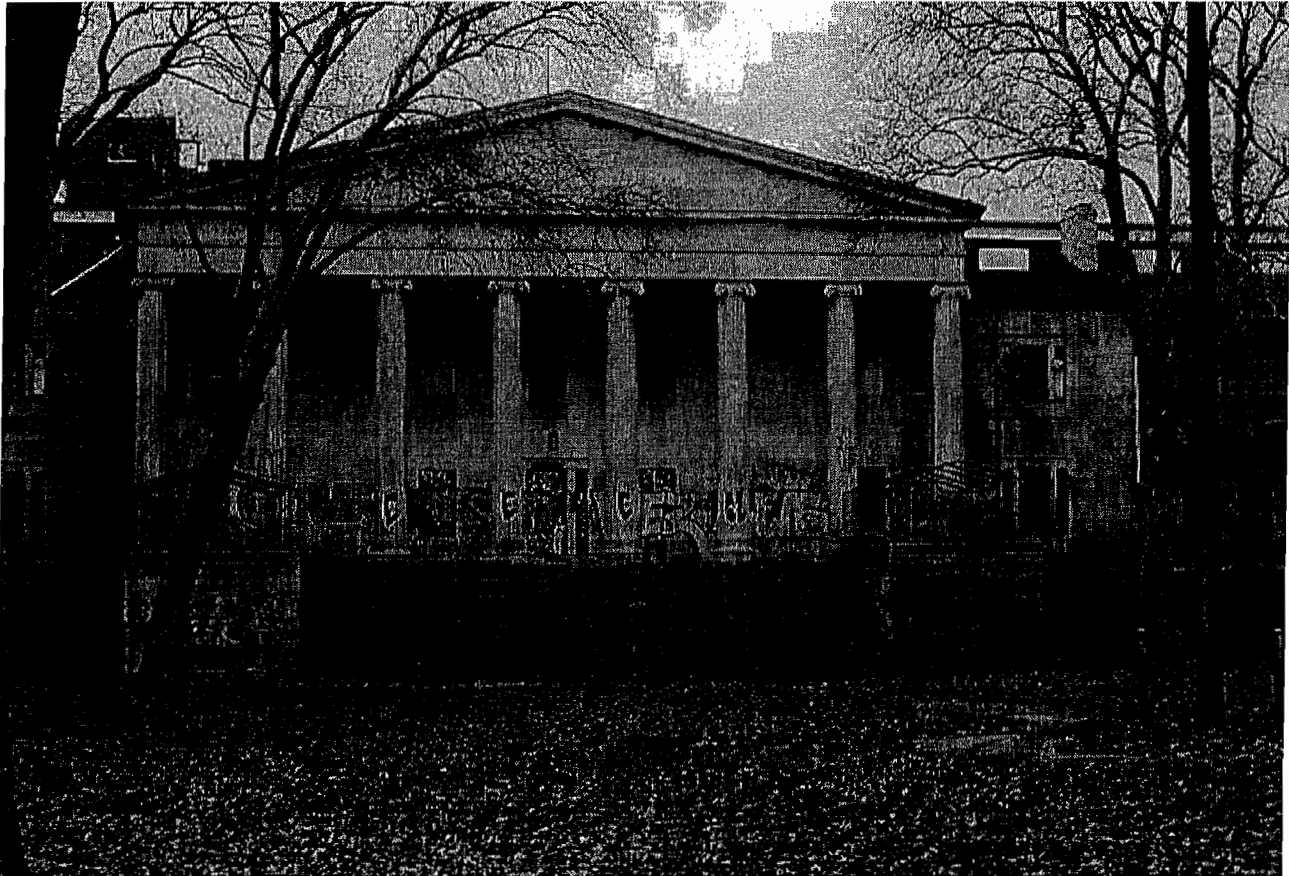
Graffiti of this magnitude are a clear indication that this site is not secure. Even before the fire, vandals entered the building and damaged the stunning cantilevered staircase flanking the chapel. (For more photos of the building past and present, see the online exhibition based on Ann Hoskins-Brown's tabletop display.)
