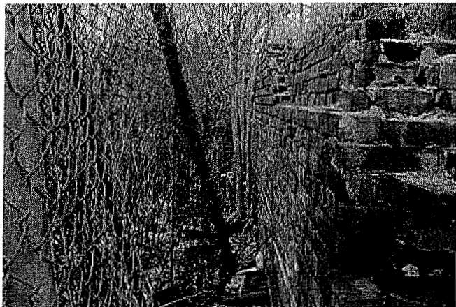
This gap in the fence behind the property is another easy entrance...
